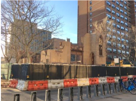
Current BHH condition (Lot 37)
